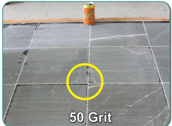
FIGURE 2-C: FLOOR AFTER 50 GRIT DIAMOND STRIPS. NOTICE IN THE YELLOW CIRCLE - THE LIPPAGE BECOMING LESS VISABLE..
