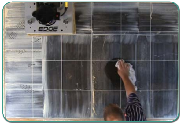
FIGURE 6-A: SPOT REMOVE THE RESIDUE TO CHECK FOR OBVIOUS FLOOR SHINE. IF NOT SATISFIED WITH RESULTS - LET SIT ON FLOOR LONGER
