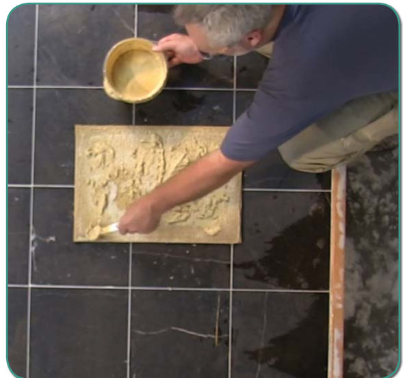
FIGURE 5-B: ALWAYS MAKE SURE TO MIX ALL OF THE PASTE UP. YOU WANT A THIN MILKSHAKE CONSISTENCY.
