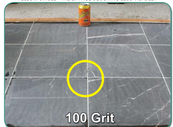
FIGURE 2-D: FLOOR AFTER 100 GRIT DIAMOND STRIPS. NOTICE IN THE YELLOW CIRCLE - THE LIPPAGE BECOMING LESS VISABLE..
