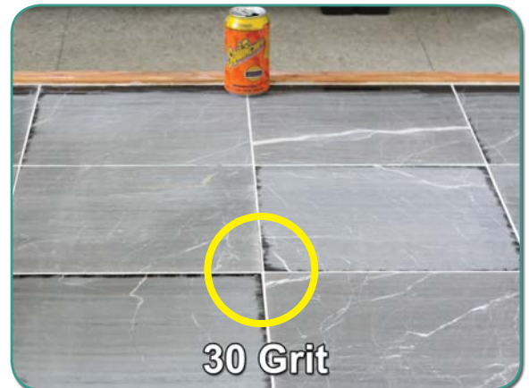
FIGURE 2-B: FLOOR AFTER 30 GRIT DIAMOND STRIPS. NOTICE IN THE YELLOW CIRCLE THE LIPPAGE OF UNEVENNESS THAT IS NOW VISABLE
