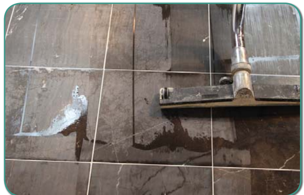
FIGURE 1-B: USING A VAC WAND TOOL - VACUUM UP ALL SLURRY.
