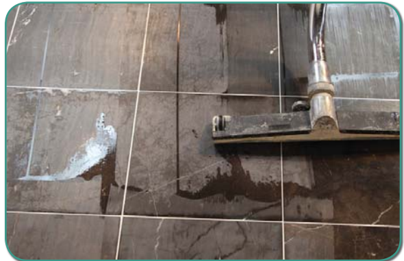
FIGURE 3-B: USING A VAC WAND TOOL - VACUUM UP ALL SLURRY.
