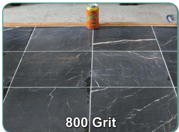
FIGURE 4-C: FLOOR AFTER 800 GRIT DIAMOND STRIPS
