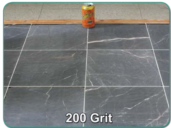
FIGURE 4-A: FLOOR AFTER 200 GRIT DIAMOND STRIPS
