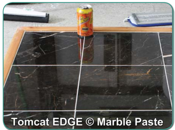
FIGURE 6-B: FLOOR AFTER MARBLE PASTE WAS UTILIZED
