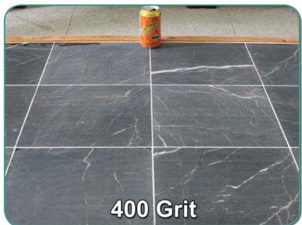
FIGURE 4-B: FLOOR AFTER 400 GRIT DIAMOND STRIPS
